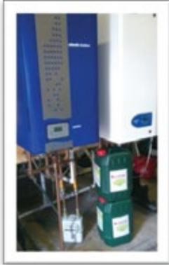
Cascade Manager with an outside ambient temperature (OAT) sensor. Direct Hot Water Supply (DHWS) is delivered by separate gas-fired Hamworthy heaters and this
