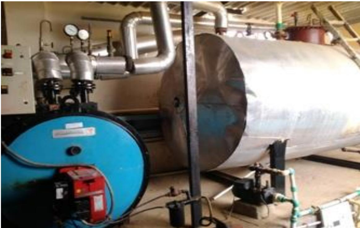
Hot water generated per HSD with water was 724.1 Litres. So it consumed 135 Litres HSD to generate 98000 Liters of hot water. If boiler was running on water, consumption could be  $51000/724.1 = 70.4$  Litres HSD. But with Hydromx it consumed 42 Litres HSD, so the saving is  $70.4 - 42 = 28.4 / 70.4 * 100 = 40.4\%$  saving.
